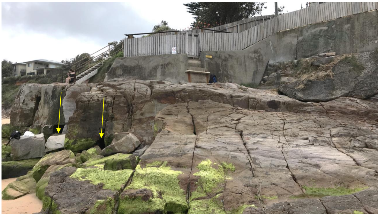
Figure 4: Examples of undercut areas (at arrows) at cliff at subject property (photograph taken 2 January 2018)
