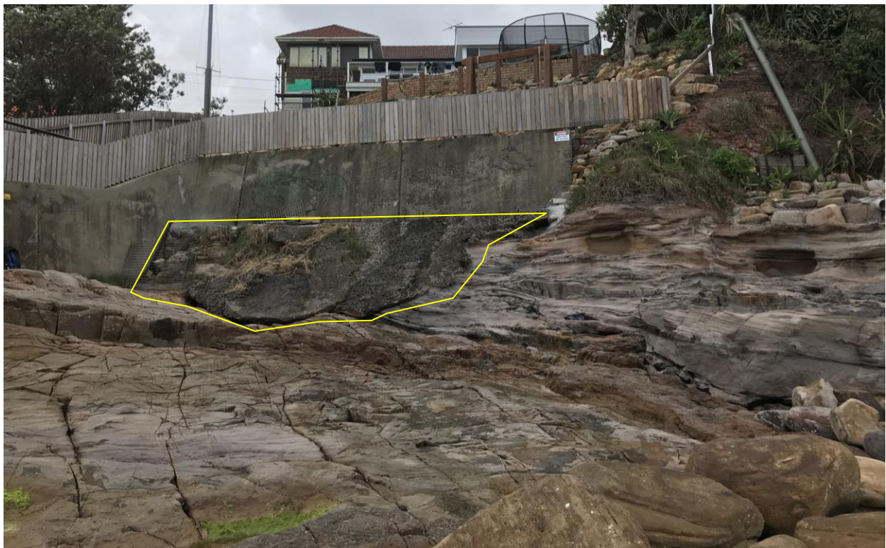
Figure 6: Existing concrete face proposed to be repaired with shotcrete and rock bolts (photograph taken 2 January 2018)
