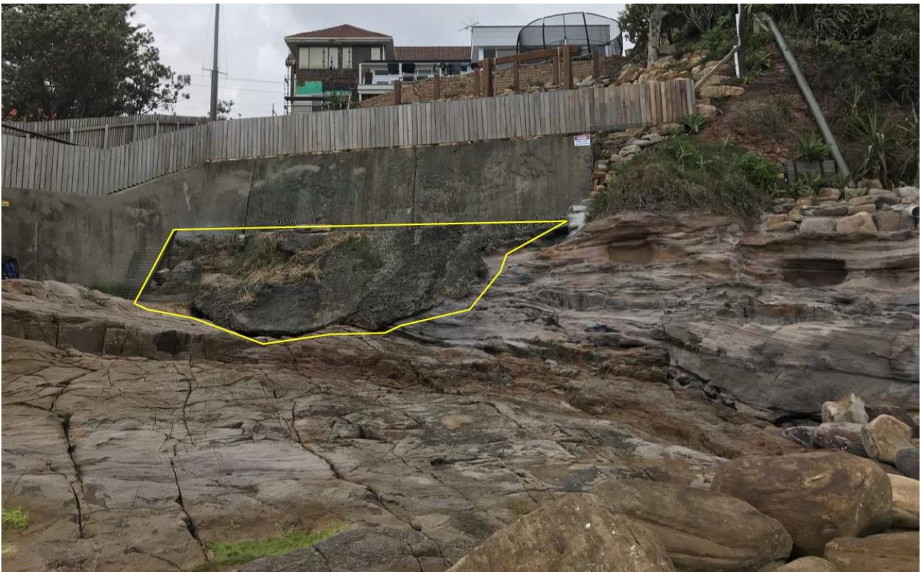
Figure 1.1 Area of concrete face requiring shotcreting and rock bolts (Horton, 2020)
